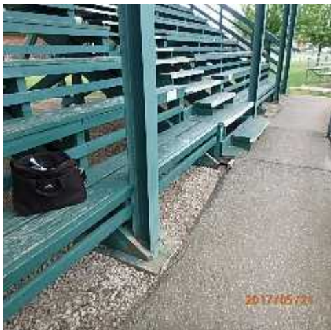
Photo 15: Steel columns at front of grandstand.
