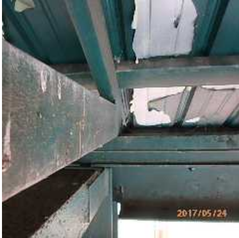
Photo 9: Purlin, truss, plate connection.
