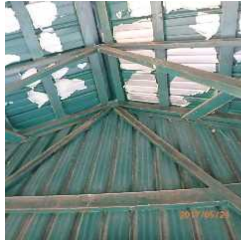
Photo 14: Typical Gable end from interior.
