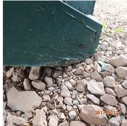
Photo 42: Stringer on buried footing.
