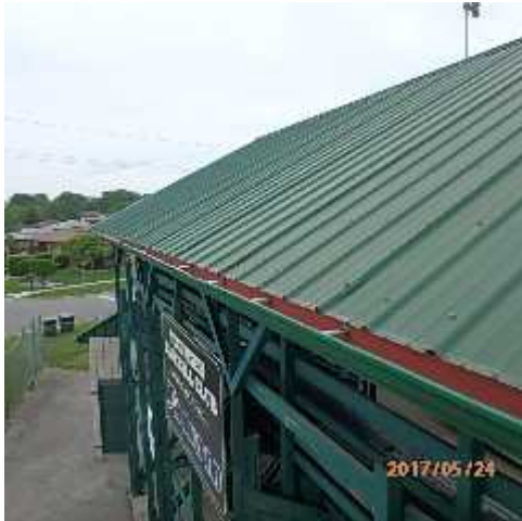
Photo 3: Typical metal roof condition.
