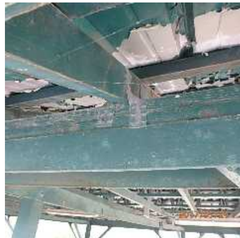
Photo 12: Perimeter hold down anchor.
