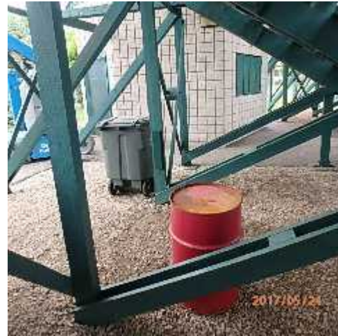
Photo 26: Stringers, posts and diagonals.
