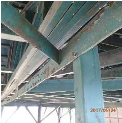
Photo 19: Diagonal bracing in horizontal plane.
