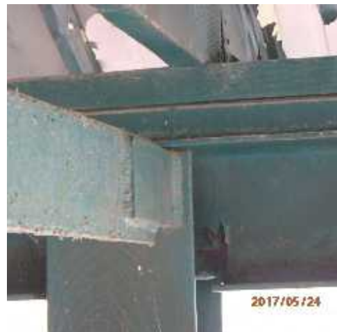
Photo 16: Front column and channel beam.
