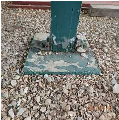
Photo 39: Typical post on footing.
