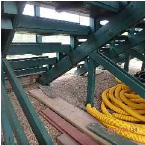
Photo 25: Stingers, posts and diagonals.
