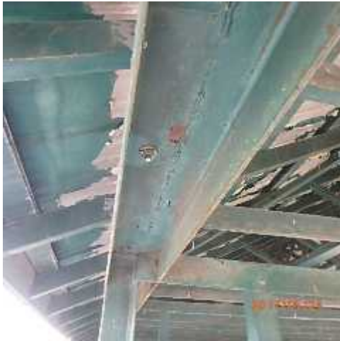
Photo 13: Perimeter steel angles.
