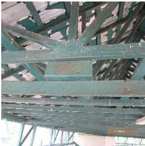
Photo 11: Gang-nail connection.
