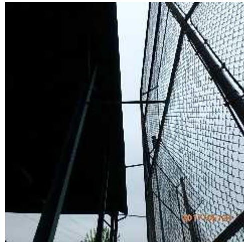
Photo 54: Backstop connection to grandstand.
