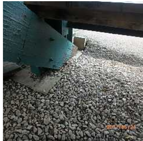
Photo 40: Typical stringer base.
