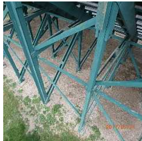
Photo 28: Typical stringer bay.
