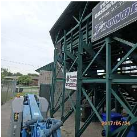
Photo 27: Bracing between stringer bays.
