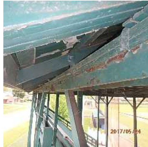
Photo 18: Steel angle between rear posts.
