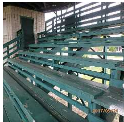
Photo 24: Floor boards and seats on stringers.
