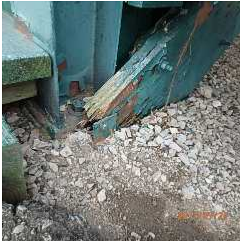
Photo 37: Typical stringer at steel column base.
