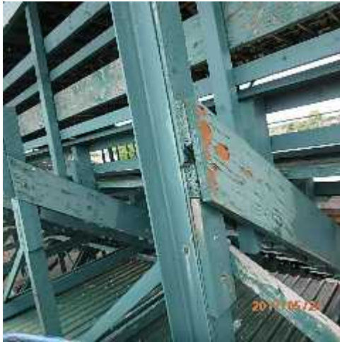
Photo 17: Steel angle and wood post.
