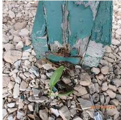
Photo 38: Post and diagonal at buried anchor.
