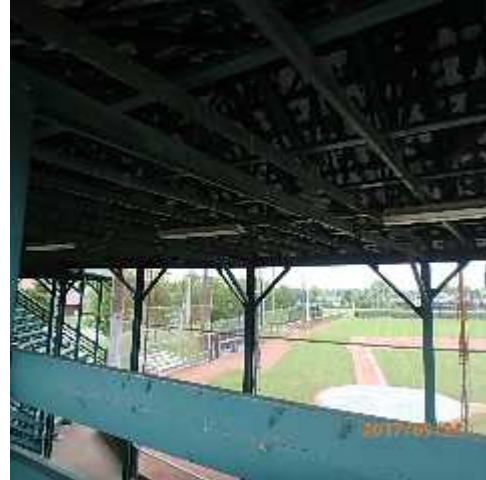
Photo 10: Typical truss layout.
