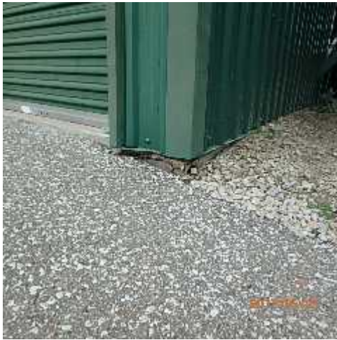
Photo 51: Storage shed on wood footing.
