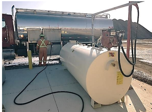
Example of above-grade fuel oil storage tank
