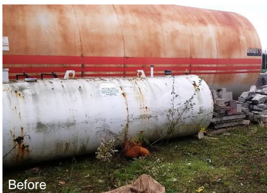
Example of above-grade fuel oil storage tank
