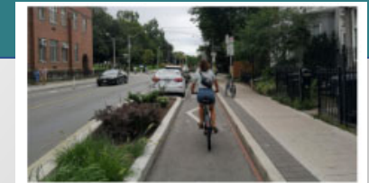
Figure 4.26 – Cast-in-place Concrete Curb Separating a One-way Separated Bicycle Lane, Toronto
