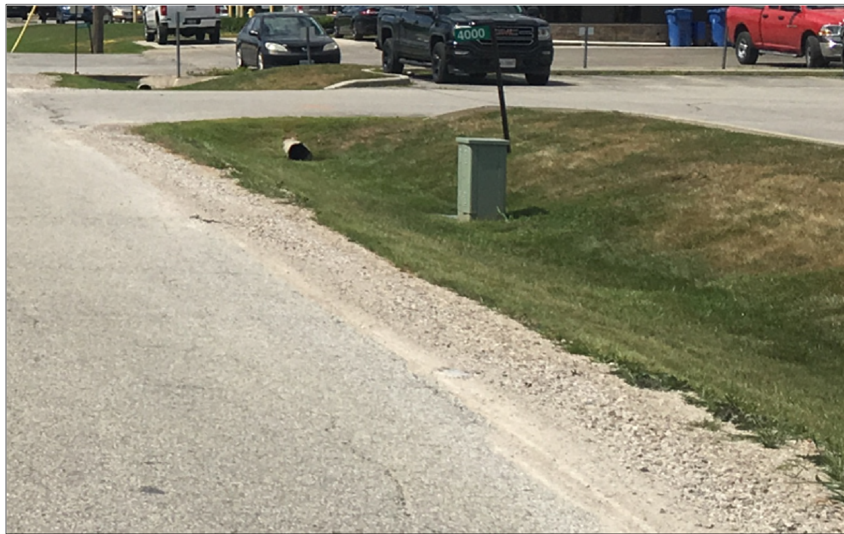
SWALE WITH DRIVEWAY CULVERT (TYPICAL)
