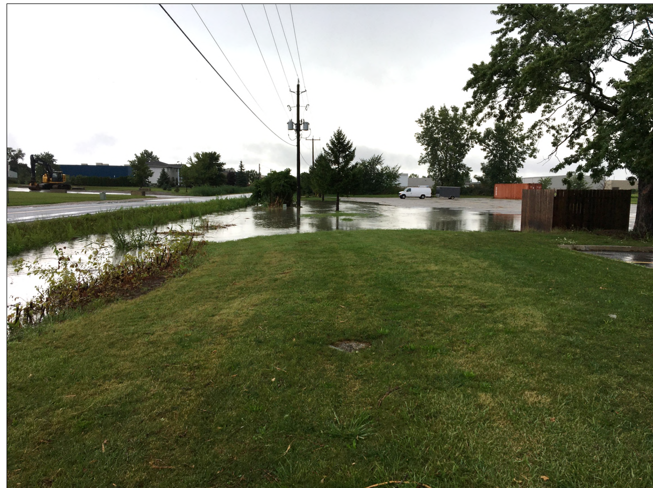
OUTER DRIVE NEAR CONNECTOR ROAD (9:20AM) WOLFE DRAIN OVERFLOW ONTO CHURCH PROPERTY
