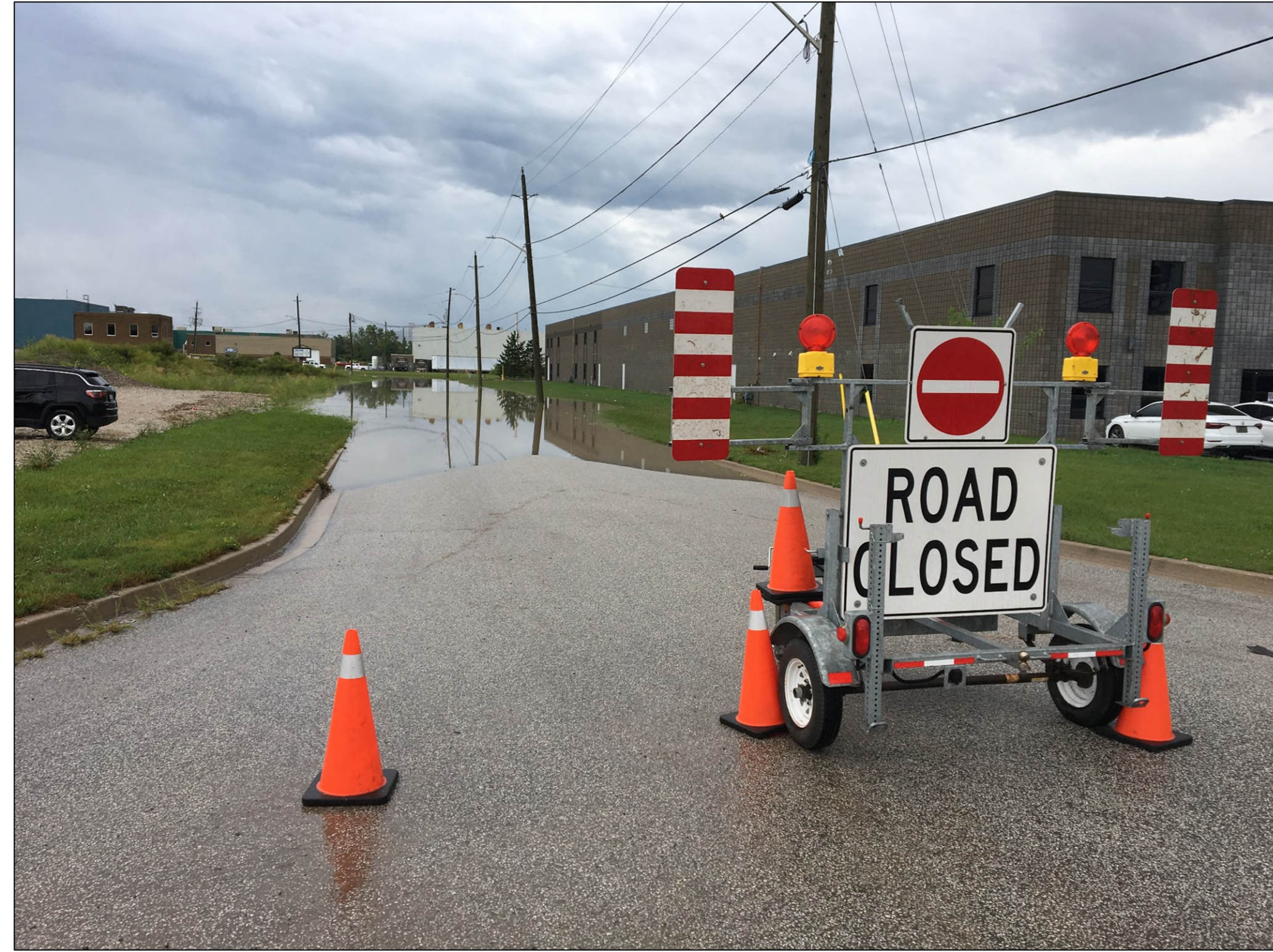
BLACKACRE DRIVE NEAR OUTER DRIVE (9:33AM) EXCESSIVE PONDING AT ROADWAY SAG
