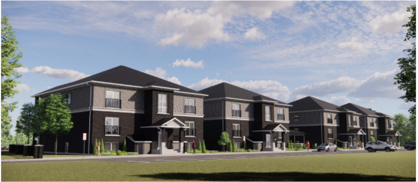
View of Rear Facade, looking southeast towards Lesperance Road
