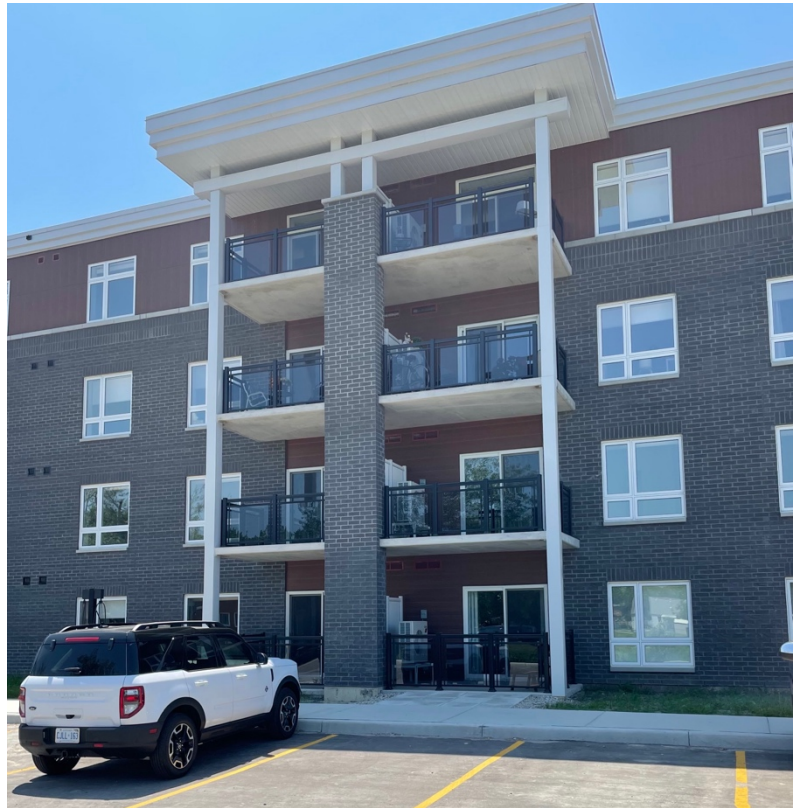
Existing 4 Storey Apartment Style Rental Building
