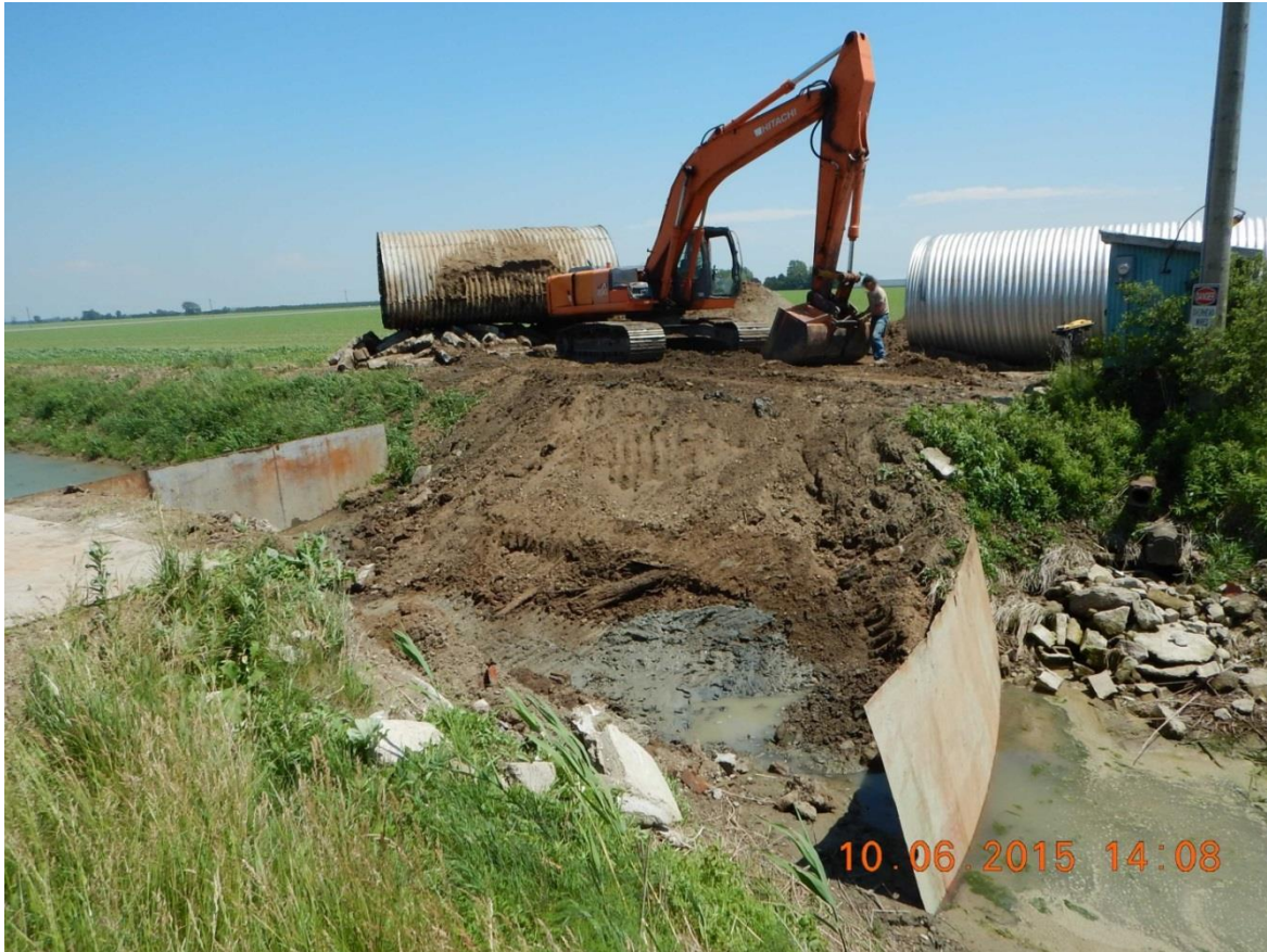
Figure 2. Isolation of Site
